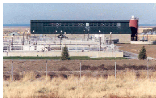
Tooele Wastewater Reclamation Plant
